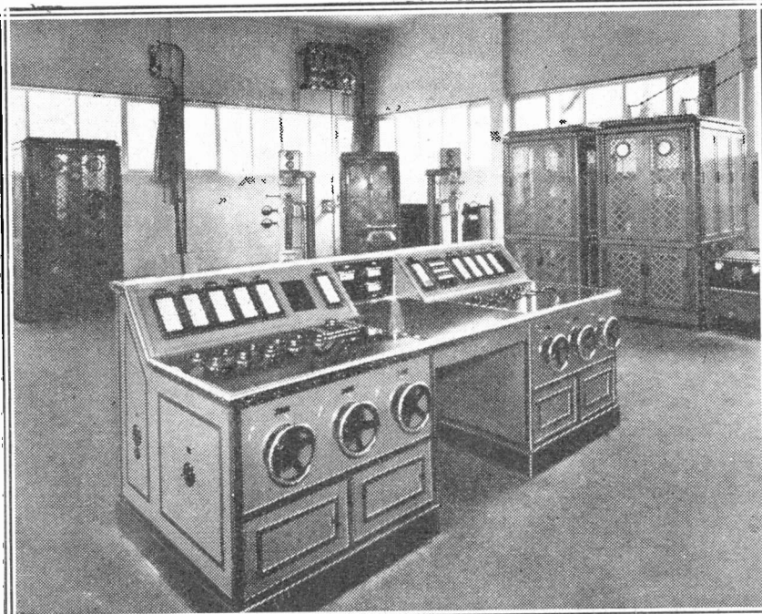
The imposing array of meters on the control desk at the Frankfurt station tells the engineer-in-charge exactly how the transmitter is working without his having to inspect each part of the apparatus.
